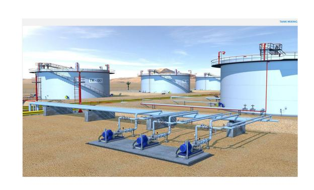
When residual water has been drained off, the crude must be thoroughly mixed before processing - this is done by either externally circulating the crude contents using a pump...
