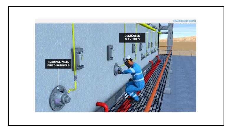
Each radiant cell has terrace-wall fired burners arranged at four levels to provide even heat distribution along the length of the radiant tubes.
