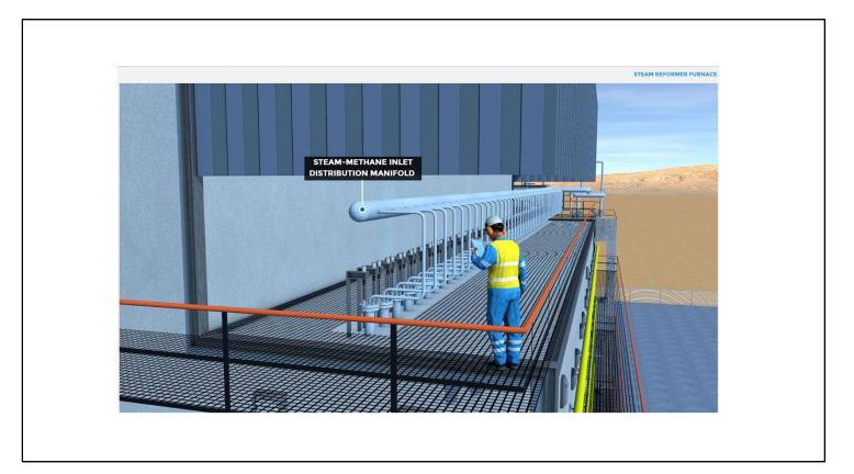
A mixture of steam and methane passes along an inlet manifold that distributes it evenly to the row of 48 radiant tubes.
