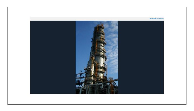
The Main Fractionator is a large tower with two side strippers.
