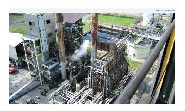
This image shows a typical cabin-type Coker Heater with a heat recovery steam generation system.
